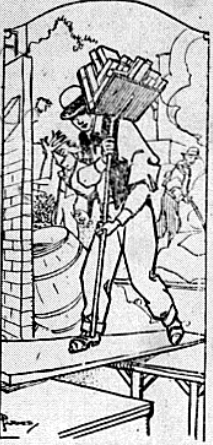
SET TO CARRYING BRICK FROM THE SIDEWALK.
