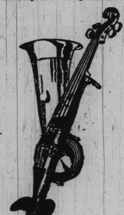
accordingly, and thus every vibration is transmitted to the diaphragm. The diaphragm sets in motion the air contained in the resonator, the resonator augmenting and distributing the same to the surrounding atmosphere.
