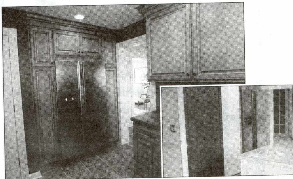
Borrowing unused space from the stairwell allowed the installation of two pantry cabinets (above, left). The space before (above).
